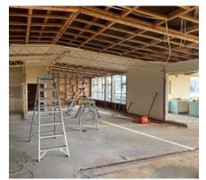
During the holidays work began on the refurbishment of the Administration block. A large amount of the demolition was done prior to Christmas, and 99% of the rest was completed during January. We are now at the point where 75% of the new framing has been erected. We are hoping to be back in the administration building early in Term 2.
